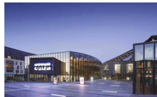
La Grande Passerelle, Saint-Malo © Architecture-Studio
